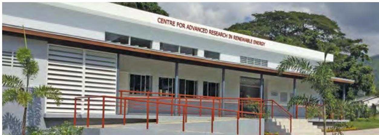
The Caribbean's first Net Zero Energy Building (NZEB) is constructed at The UWI Mona Campus.
